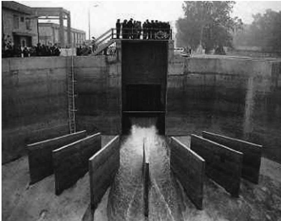
Fig. 18.10 : Water treatment plant
