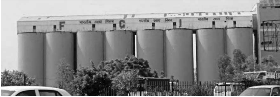
Fig. 1.10 (a) : Silos for storage of grains
