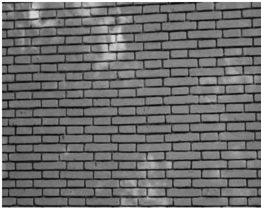
(a) Brick wall
