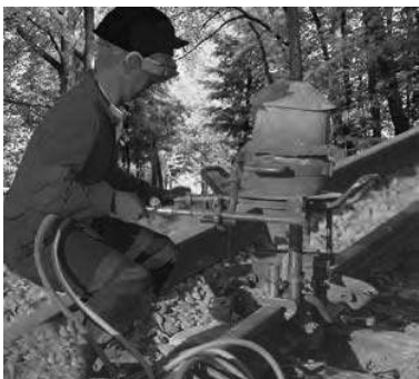
Figure 3.11 Thermit process for joining railway tracks
