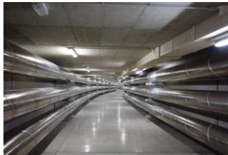
View into the tunnel with 400 m bending radius of GIL.
