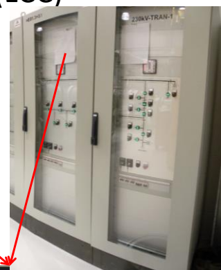
Hardwire with electromechanical relays
