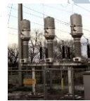
145 kV Blue Instrument Transformers 2 in operation in GER since 2018 9 ordered in NOR, SWE, GER
