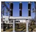
72.5 kV Blue Circuit Breakers, LT 6 in operation in FRA, LUX, DEN, AUS since 2010
