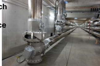
View into the tunnel from the connection shaft the overhead line.
