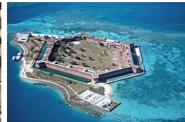
An aerial view of Fort Jefferson in Dry Tortugas National Park
